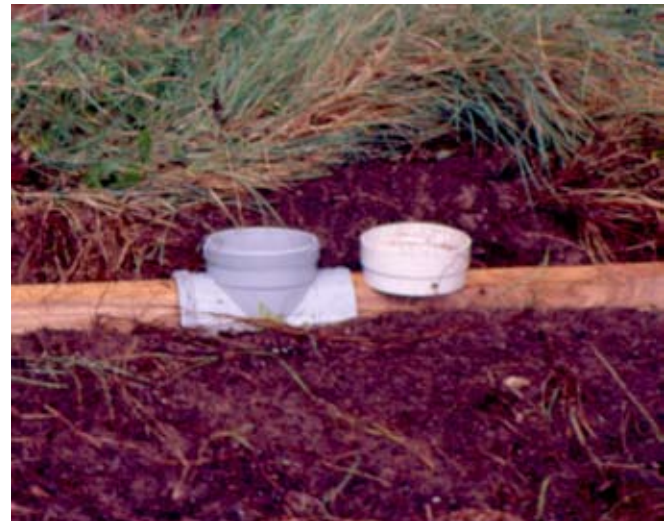
Figure 5. Installing a termite aggregation station with plastic T piece and timber.
