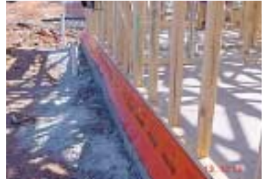
Kordon TB with timber frames in place
