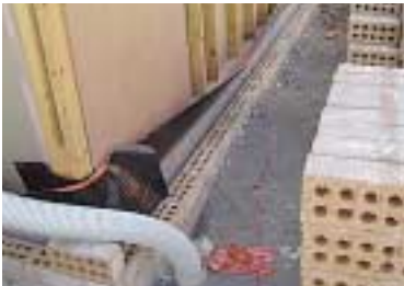
3 & 4, Kordon TB pinned to frame whilst bricks are layed to Damp Proof Course level
