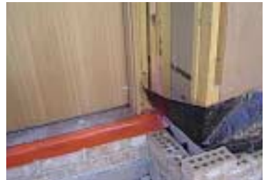
5 & 6, Kordon TB secured to outer brick edge with spray adhesive/doubs
