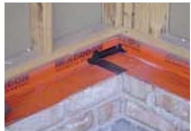
7 & 8, external, internal corners, overlapped, folded, secured with spray adhesive and cloth tape.
