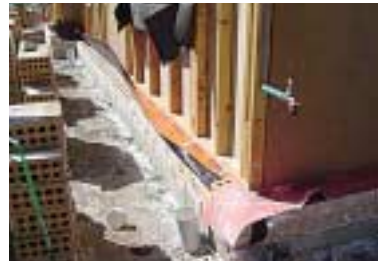
3 & 4, Kordon TB pinned to frame whilst bricks are layed to Damp Proof Course level
