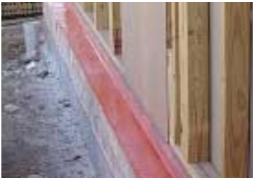
5 & 6, Kordon TB secured to outer brick edge with spray adhesive/doubs
