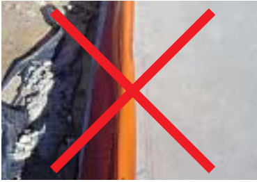
incorrect installation - Kordon TB not installed to frame chalk line
