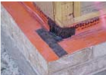
7 & 8, external, internal corners, overlapped, folded, secured with spray adhesive and cloth tape.
