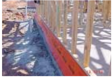
Kordon TB with timber frames in place
