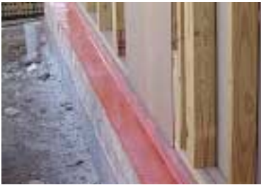
5 & 6, Kordon TB secured to outer brick edge with spray adhesive/clouts
