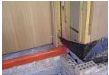
5 & 6, Kordon TB secured to outer brick edge with spray adhesive/clouts
