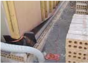
3 & 4, Kordon TB pinned to frame whilst bricks are laid to Damp Proof Course level
