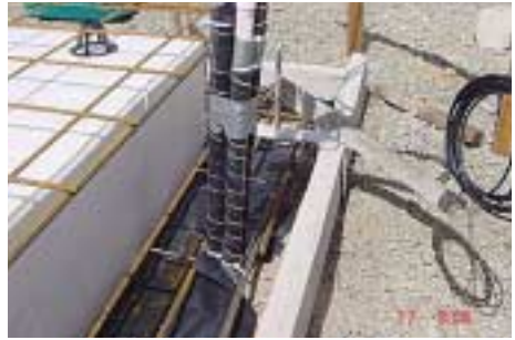
photo 2 showing multiple pipes each protected with Kordon
