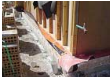
3 & 4, Kordon TB pinned to frame whilst bricks are laid to Damp Proof Course level
